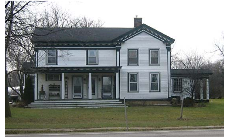
Loren Woodard House 927 East Grant Highway
