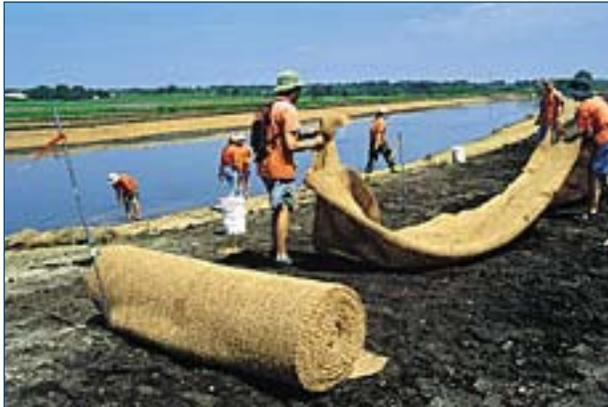
*The restoration of Nippersink Creek provides a model for re-meandering, streambank stabilization, and use of native vegetation buffer strips to improve water quality and restore habitat.*
